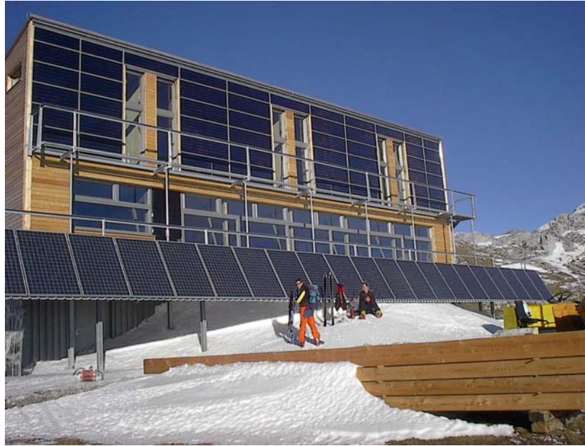
Figure 2 The “Schiestl Haus”, a prototype of an ecologically friendly alpine hut (Picture courtesy ATB Becker)
