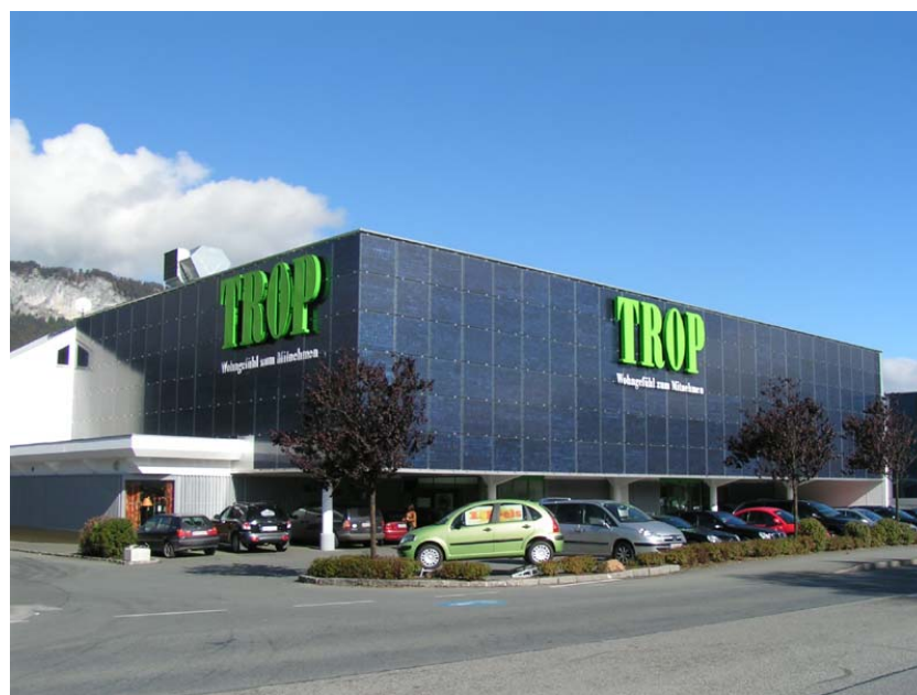
Figure 1 PV façade at a refurbished furniture store (Picture courtesy ATB Becker)
