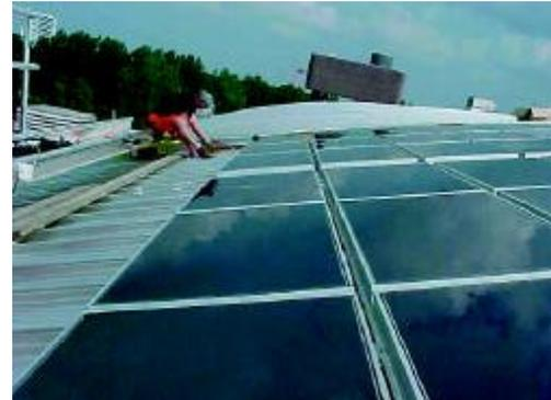
The installation comprises 7272 amorphous modules mounted on an 11 000 m<sup>2</sup> KalZip-Corus aluminium roof as part of WLD's renovation of the roof of its salt-water and fresh-water research hall.
