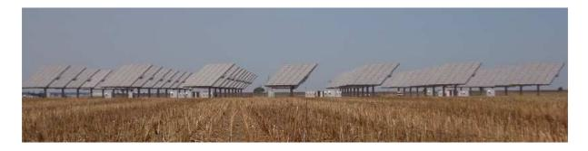
Figure 17 High Concentration PV plant (1.5 MW) installed in Écija (Sevilla), with 60 trackers
