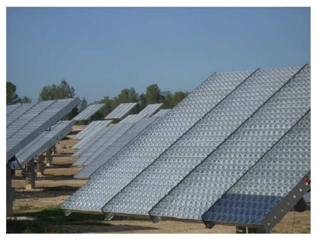
Figure 19 High concentration photovoltaic plant (800 kW) in Flix (Tarragona)
