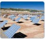
Figure 20 High Concentration PV plant (200 kW) installed in Puertollano for the Institute of Concentration Photovoltaic Systems (ISFOC)
