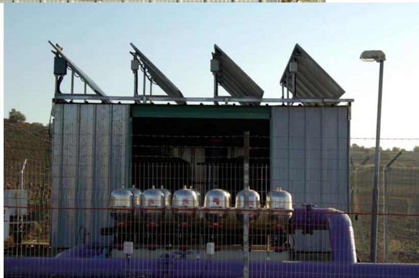
1500W PV system installed in late 2006 at a large water control station. PV in water supply and irrigation control are widespread applications of PV here (Photo credit: Interdan Ltd.)
