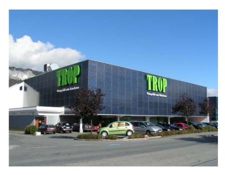
Figure 1 PV façade at a refurbished furniture store (Picture courtesy ATB Becker)
