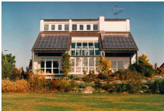
Figure 7: Winner of the competition “Most Attractive 1000-Roofs-PV system” (Bechtold).
