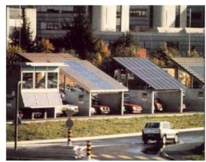
**fig** 5 Three of the Demosite pavilions, demonstrating different PV roof integration systems
