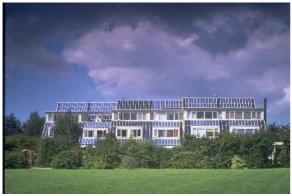
fig. 1 Integrating PV into existing dwellings (picture courtesy R.Schropp; project Bear Architects)
