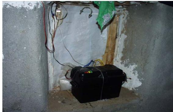
**Figure 3:** Poorly installed PV system
