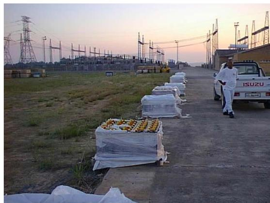
**Figure 1:** Incorrect storage of batteries
