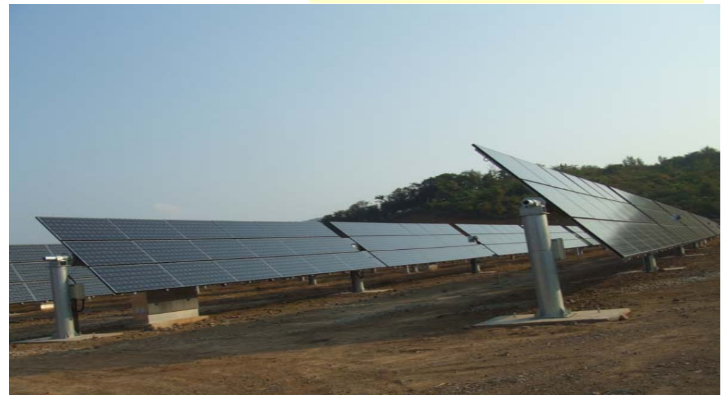
Gohung, 1.5MW, 1 axis, 2006
