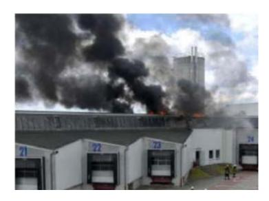
Hot spot effect leading to local failure Fire disaster of Buerstadt PV station in Germany, June.2009
