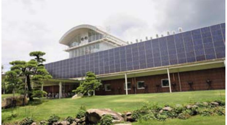
*This 40 kW facade is part of a 480 kW system installed at Saishunkan Hilltop Yakusai Factory Park under the Advanced PV Field Test. [PHOTO RTS CORP]*
