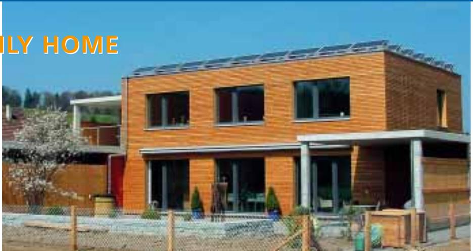
***PV, solar water heaters, a ground-source heatpump and sensible passive solar design have been combined to create an energy neutral house in Dintikon, Switzerland.***
