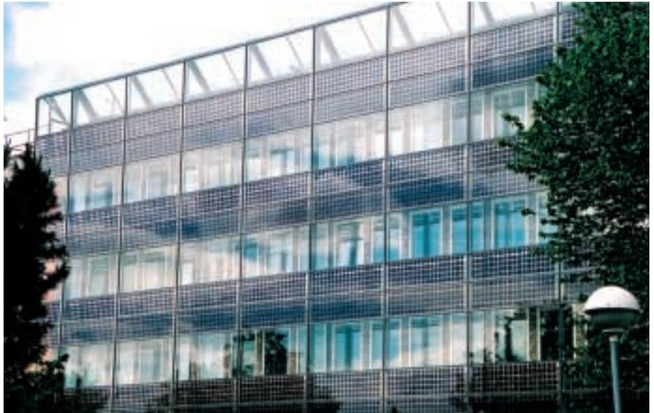
The solar skin combines two contemporary building concepts; the use of double façades in renovation projects, and building integrated photovoltaics (BIPV).
