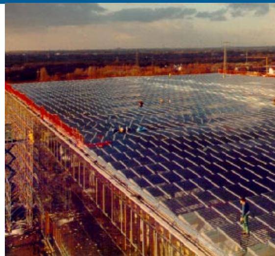
modules with differing densities of solar cells and glass of various degrees of transparency. The number of cells per module ranges between 260 and 128 (with corresponding power outputs of between 419 and 250 Wp) from the roof areas above the inner buildings to the middle and edges of
