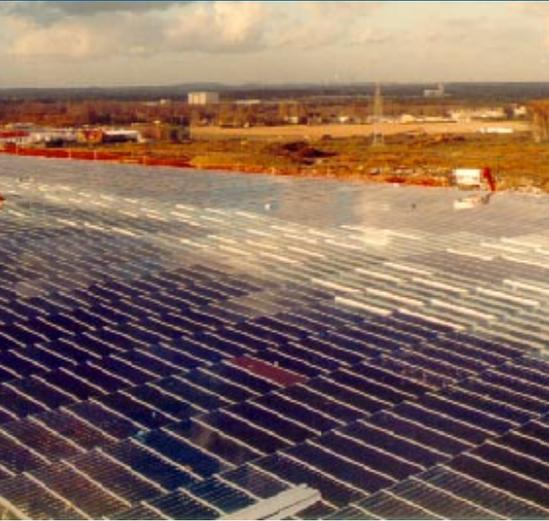
the roof where more daylight is needed. The inverter concept is innovative for a project of this size. 569 String inverters are used in order to reach the highest system efficiency for the complicated module distribution on the roof. Installation of the inverters only took about three months in to-
