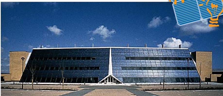
***Doxford's 'Solar Office', designed by Studio E Architects is the first speculatively constructed building to integrate photovoltaic technology.***
