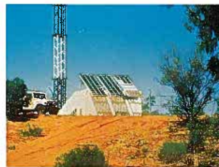
Telstra Microwave Repeater Station, Central Australia. [COURTESY TELSTRA]
