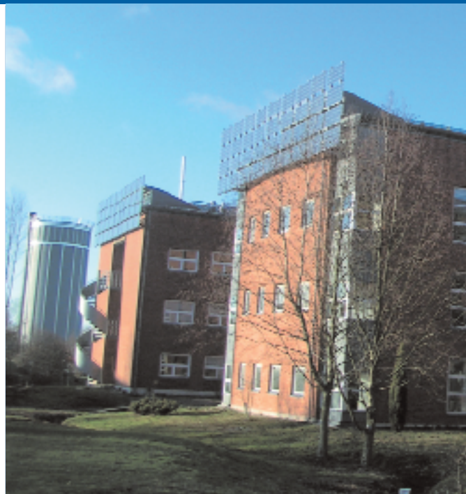
Fig. 1 – A total of 109 kWp has been installed on the roof and on the facade, as well as above the windows as sunscreens at the House of Ecology, Lund University. The different parts of the system demonstrate different ways of PV architectural integration.
