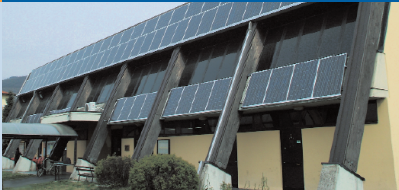
Fig. 2 - Building integrated 13 kW PV plant, Gavardo (BS) (photo GSE).
