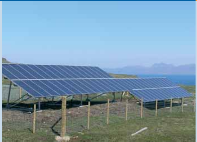
Fig. 3 - This 9,9kW array was installed during 2007 as part of the Isle of Eigg Electrification project (photo Wind and Sun).
