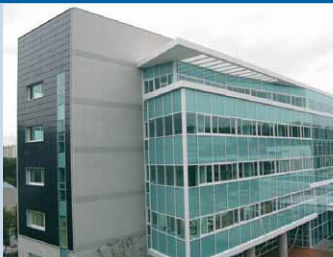
Fig. 1 - The 13 kW grid-connected BIPV systems installed on the KIER research building in 2007.
