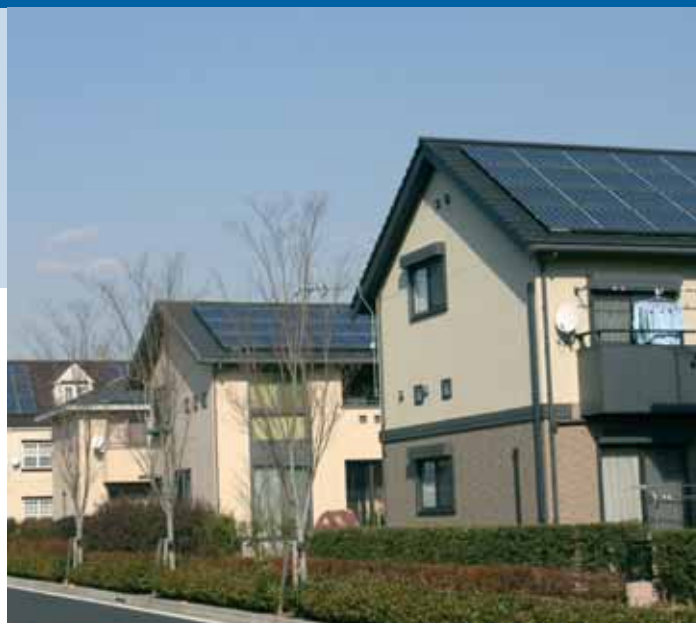
Fig. 5 - Intensively installed PV system for houses, Pal Town Jyosai-no-Mori, Total 2 130 kW, 553 houses (Average: 3.85 kW per house, Ota City, Gunma Prefecture (photo Otacity Land Development Corporation).
