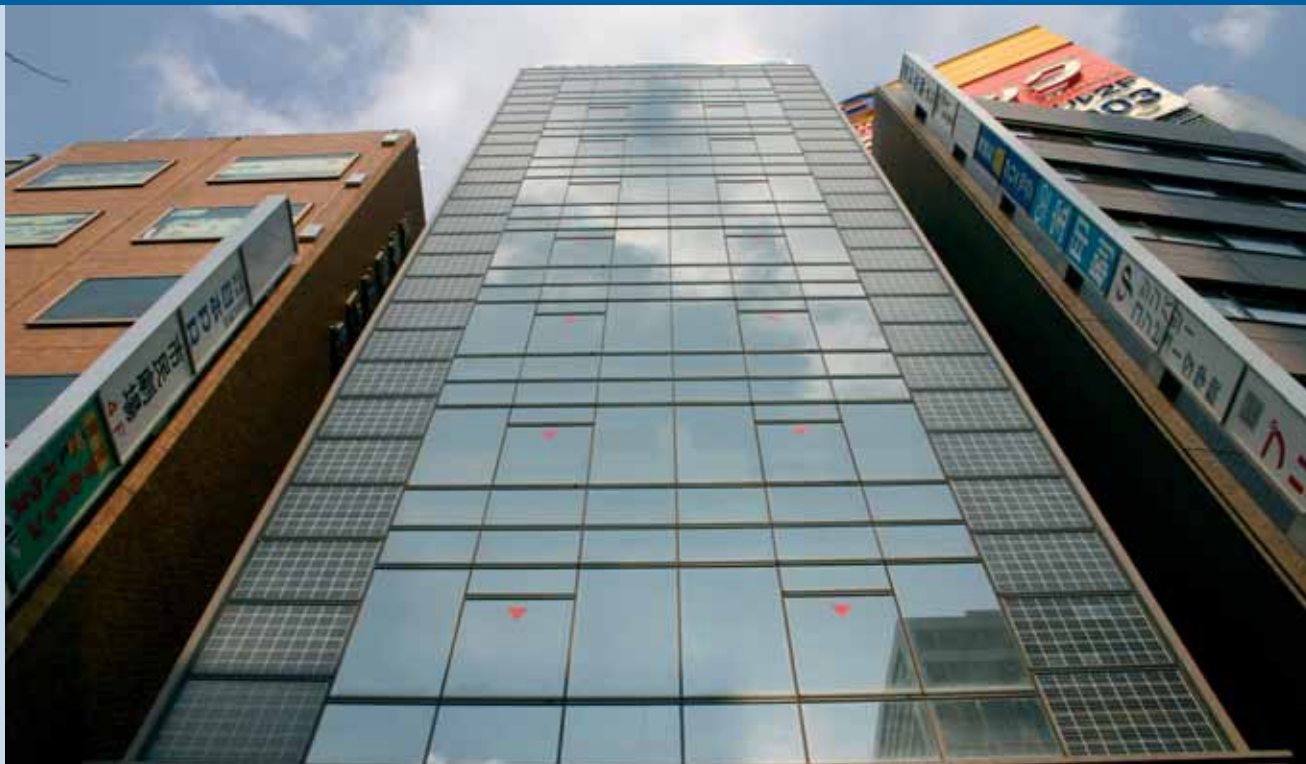
Fig. 4 - GG Solar Building, 10 kW, Chuo-ku, Fukuoka City (photo RTS Corporation).
